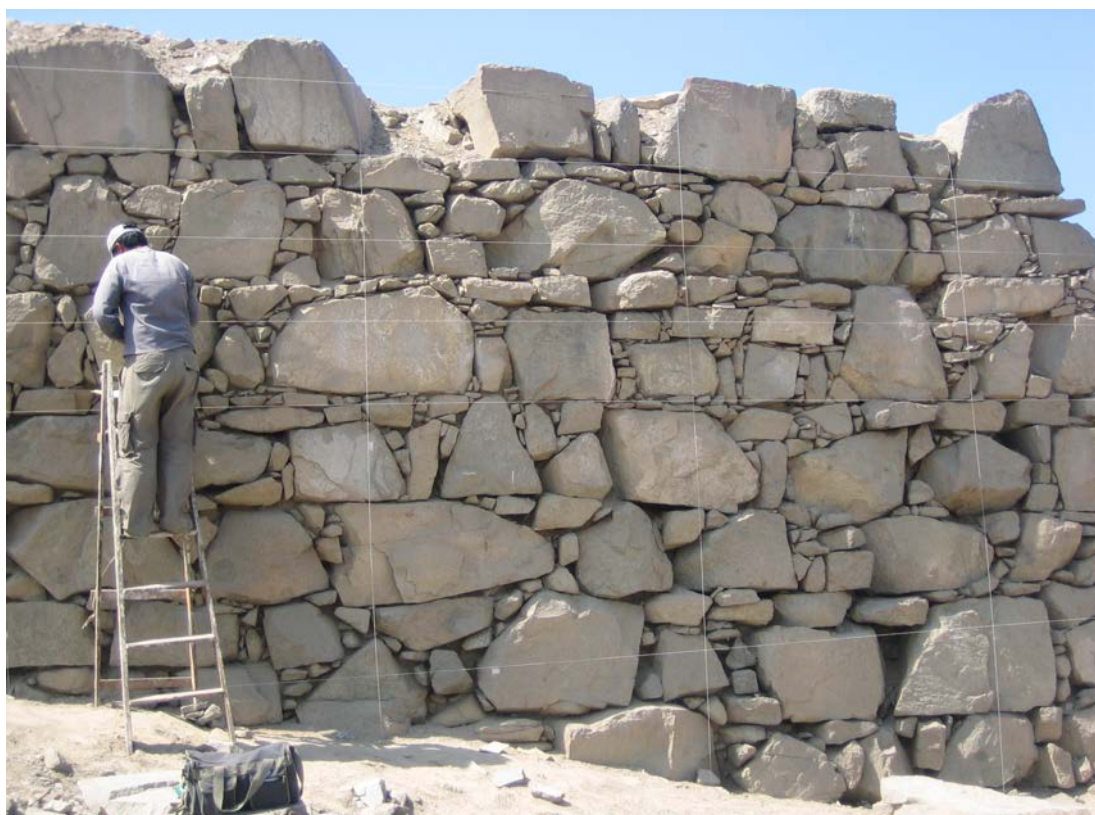
Figura 6. Detalle del muro norte de la EA 1. Detail of the North wall of EA 1.
